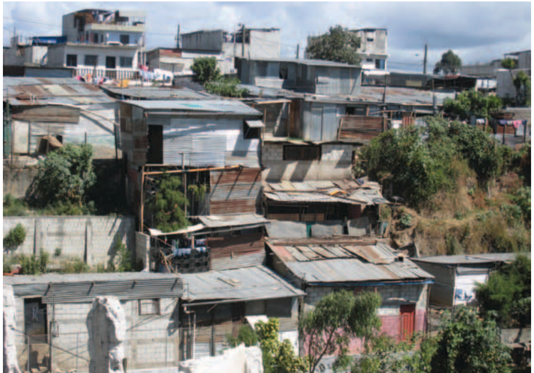
Improvised housing offers an alternative but inadequate option for low-income families in Villa Nueva, Guatemala.
